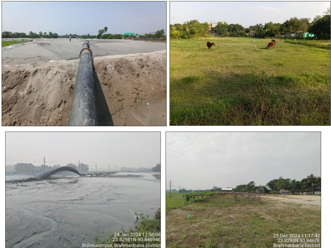
Figure 4: Dyke 26 at River Route-09 Before (Low Land: One Crop: Rice), After (High Land: Agricultural Practices for Two Crops, Pasture Land etc.)
