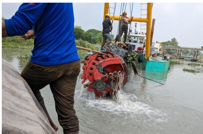
Figure 12: Lot 2, Route-09. (Bancharampur-Homna Loop), Solimganj, being dredged by Cutter suction Dredger Karnafuly-07
