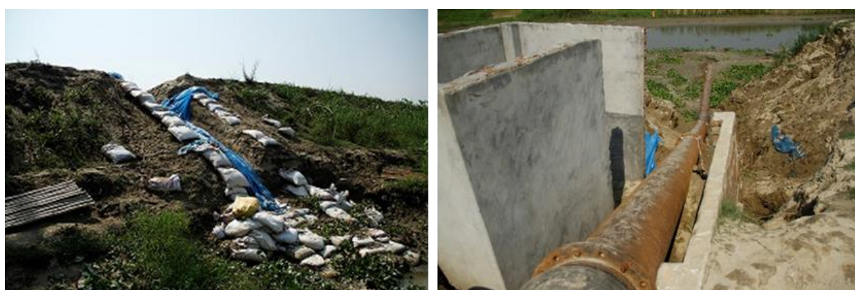
Figure 3: Dykes constructed along the river bank. Disposal of dredged materials are not maintained properly which caused breaches of the dykes and affecting the river bank
